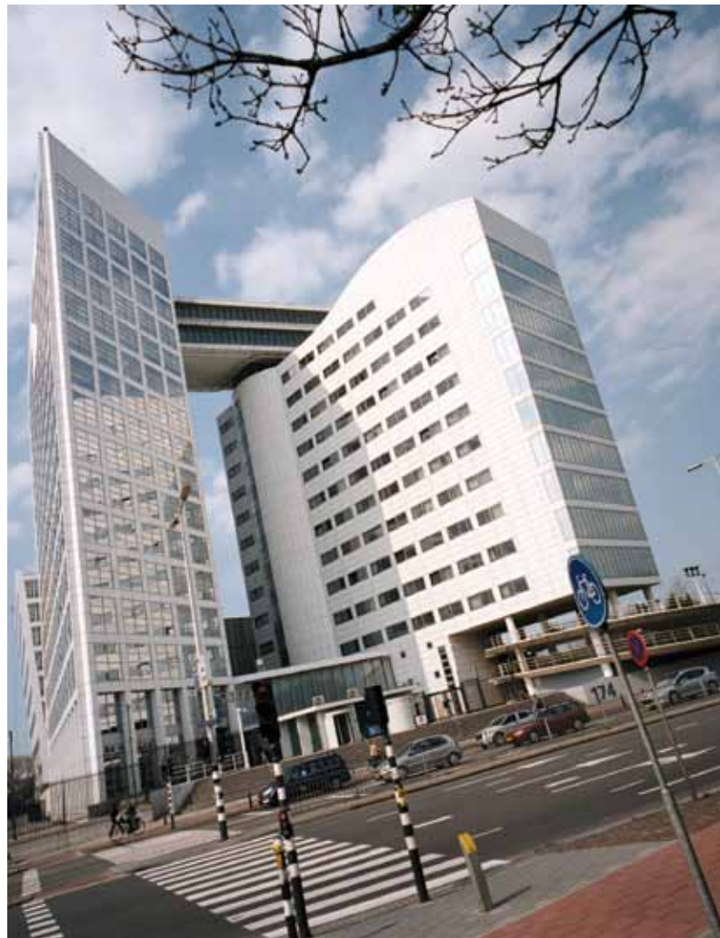
ICC Building. The Hague, Netherlands. © ICC-CPI/Max Koot
